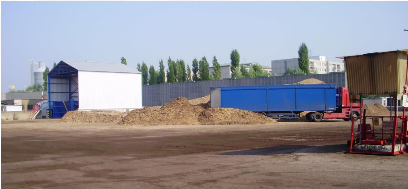
Biomass unloading yard
