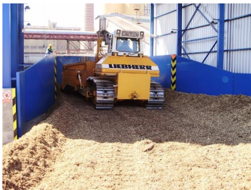
Biomass receiving area with underground screw conveyors
