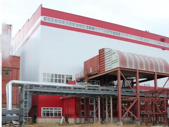
Heating plant view
