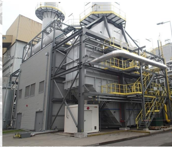
Hot water heat recovery
