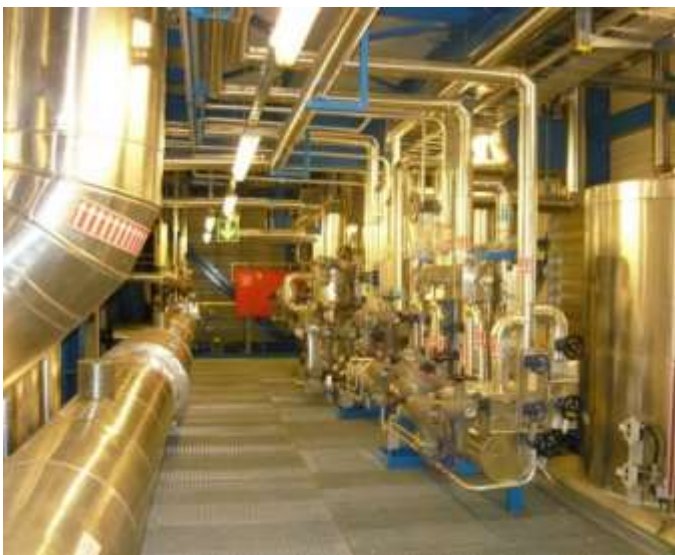
Boiler house in-view
